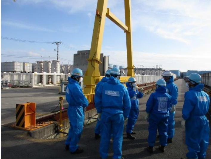
Spent adsorption vessel temporary storage
